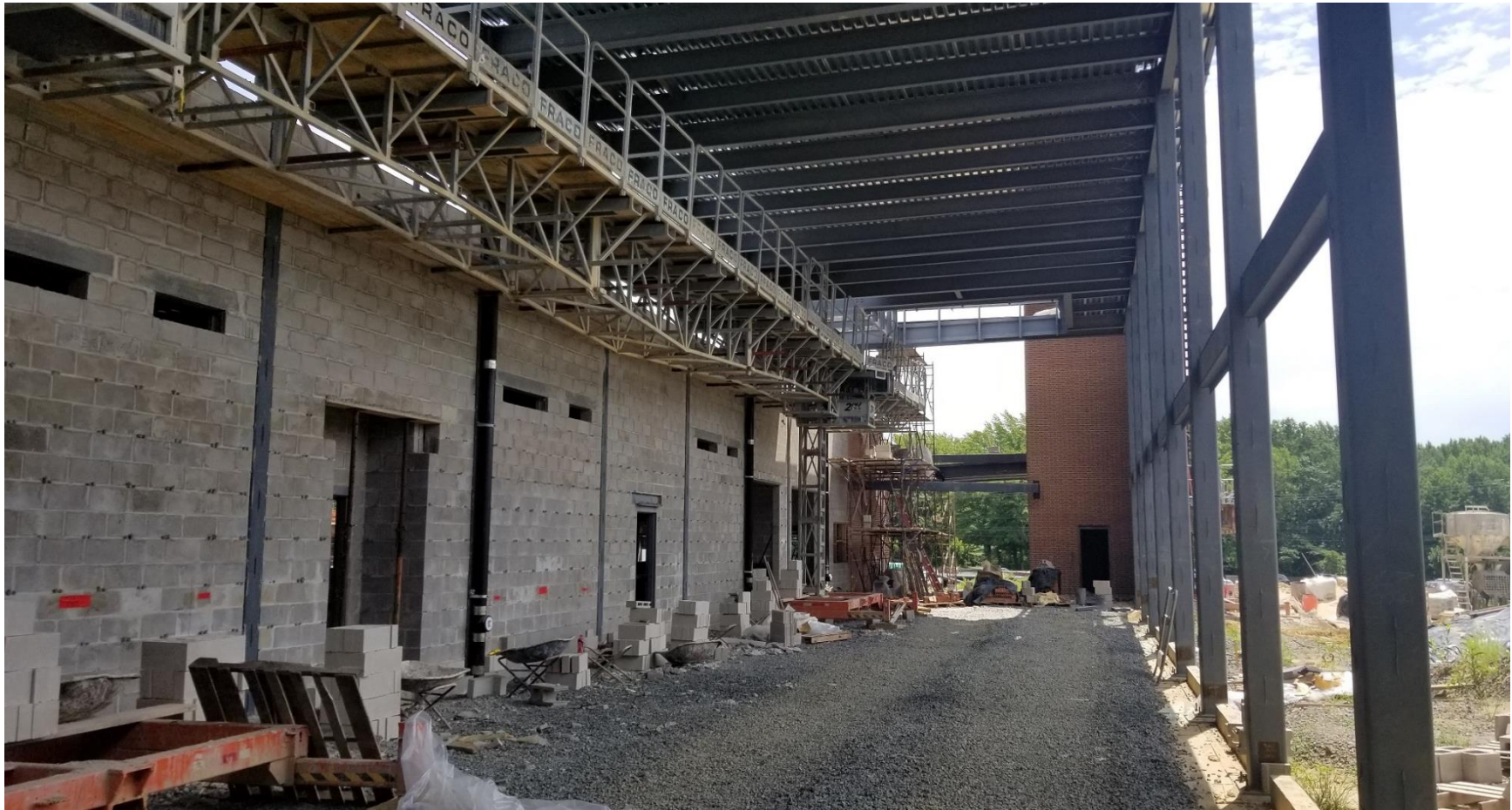
Entrance Corridor at Main Addition (Looking South)
