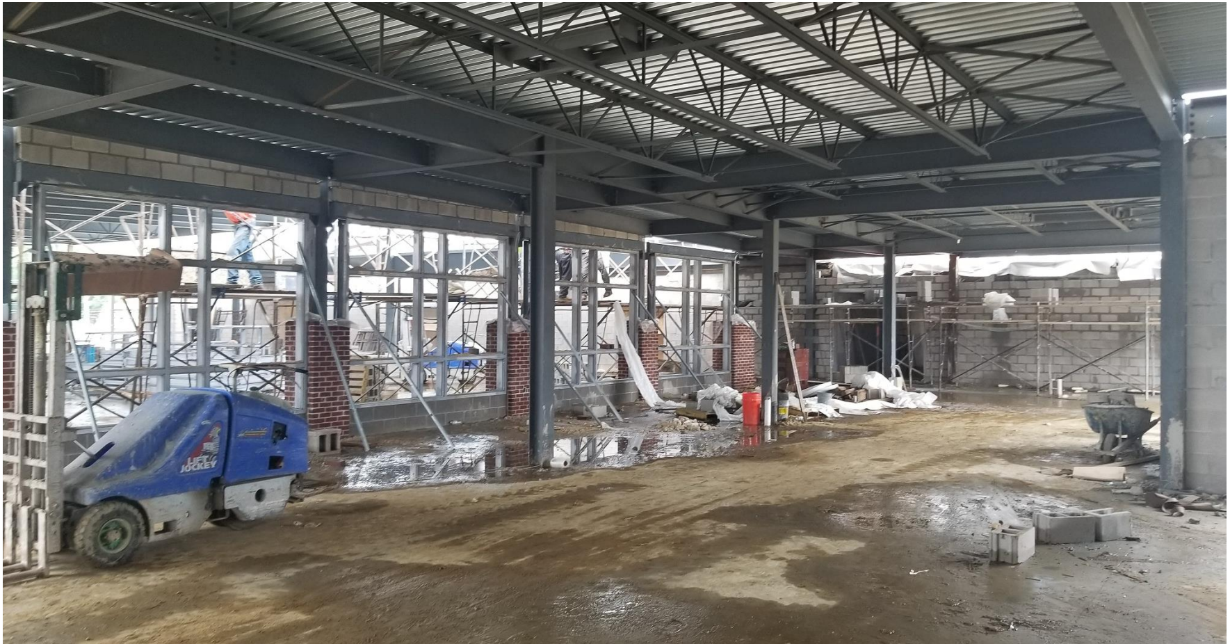
Corridor Wall at School Store in Main Addition
