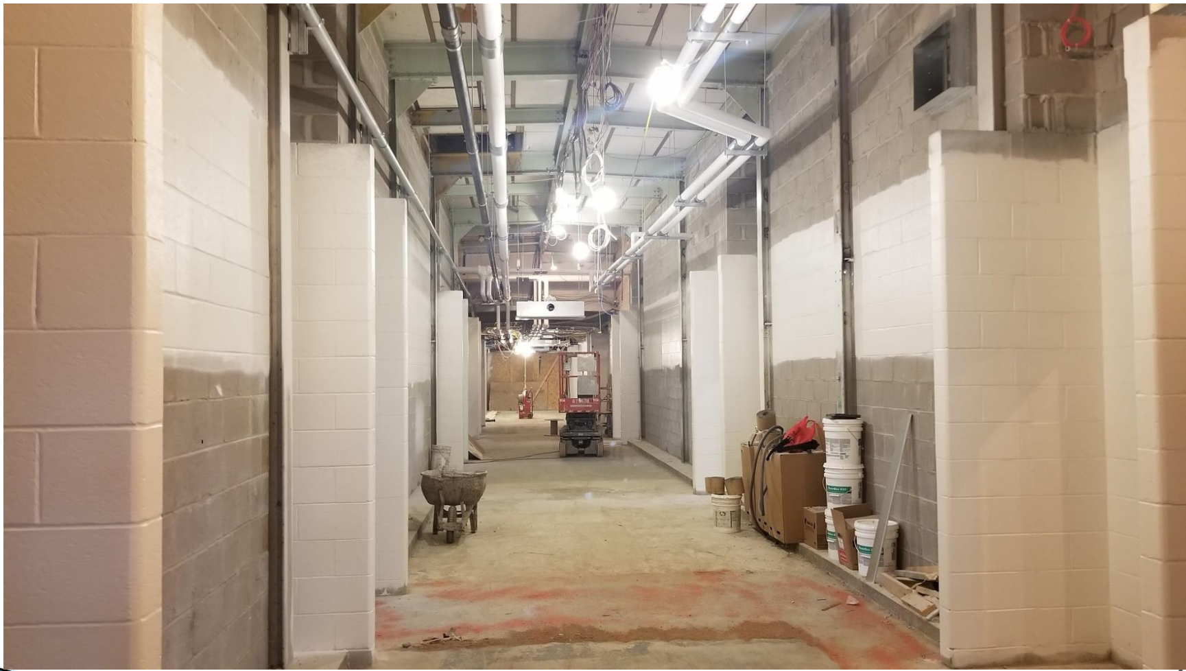
100 Wing Corridor (Old Shops Area)
