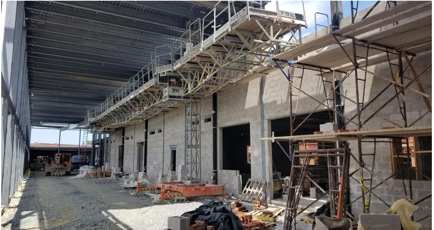
Entrance Corridor at Main Addition (Looking North)
